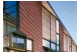
Production and office building, Baar, CH Burkart, City of Baar Building Department Baar; Barkow Leibinger Architekten, Berlin Gebr. Baur AG, Baar TECU® Oxid
