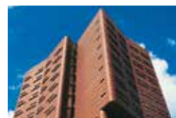
Officer's quarters of the Royal Marines of the Netherlands, Den Helder, NL Van Herk & de Kleijn Architecten BV, Amsterdam Ridder BV, Hoorn TECU® Classic
