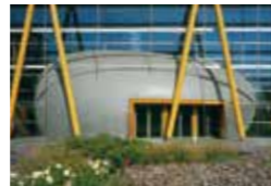
Administrative building of WeberHaus, Rheinau/Linx, D Dipl.-Ing. Günter Hermann, Stuttgart Wittenauer GmbH, Sasbach TECU® Zinn
