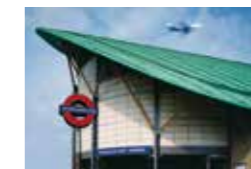
Underground station Hounslow West, London, GB Michael Watkins (Partner), London, (Acanthus, Lawrence and Wrightson Architects) Broderick Structures Ltd., Woking TECU® Patina
