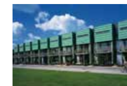
Residential building, Purmerend, NL Roy Gelders Architecten, Amsterdam Ridder Dak- en Wandsystemen BV, Hoorn TECU® Patina
