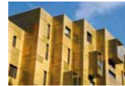
Walpole house, London, UK Make Architects, London CGL Systems Ltd, London TECU® Brass
