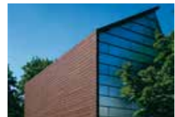
University Stuttgart, Stuttgart, D Rolf Loew, Stuttgart Dangel GmbH, Lenningen TECU® Oxid
