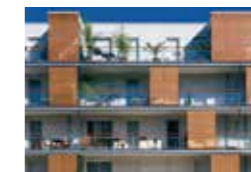
Residential Building "Le Galilée", Rennes, F Chouzenoux et Associés, Rennes SABM, Guichen TECU® Classic_mesh
