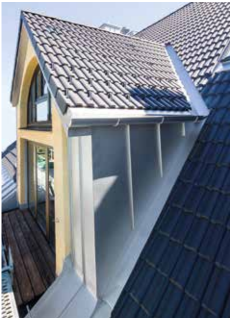
Roofinox Classic, dormer cladding and drainage, duplex, Munich, Germany
