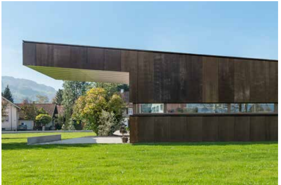
Roofinox Proton, rainscreen cladding, single family home, Vorarlberg, Austria
