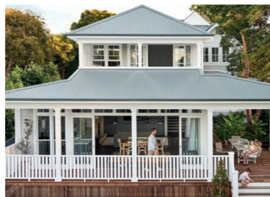
• Roofing and gutters | COLORBOND® steel Windspray® in a Classic finish.
