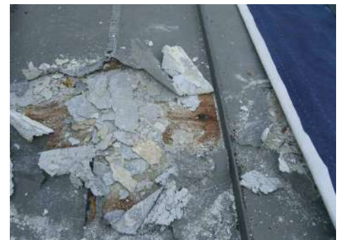
Result of using a hybrid roof
