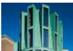
"Boscotondo", Helmond, NL Adolfo Natalini Architetti, Florence Architectenburo C. Schrauwen, Amsterdam Crombach Dakafwerking BV, Wittem TECU® Patina
