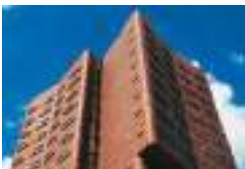
Officer's quarters of the Royal Marines of the Netherlands, Den Helder, NL Van Herk & de Kleijn Architecten BV, Amsterdam Ridder BV, Hoorn TECU® Classic
