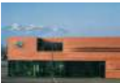
Offices and industrial building, Koblach, A AIX Architects, Feldkirch Peter GesMBH + CoKG, Koblach TECU® Classic
