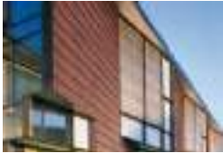
Production and office building, Baar, CH Burkart, City of Baar Building Department Baar; Barkow Leibinger Architects, Berlin Gebr. Baur AG, Baar TECU® Oxid
