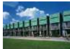
Residential building, Purmerend, NL Roy Gelders Architecten, Amsterdam Ridder Dak- en Wandsystemen BV, Hoorn TECU® Patina
