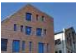
Granary Wharf - Abbey Road, Barking, UK Pollard Thomas Edwards Architects (PTE), London, UK Roles Broderick Roofing Ltd, Chobham, UK TECU® Bronze
